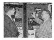
FM'S FUTURE looks bright to C. A. Priest, engineer of the General Electric transmitter department (right), and D. E. Chambers, as-sistant engineer, as they inspect one of the new GE 1 kw. FM transmitters on the test floor at Schenectady. This view indicates the basis of GE's claim that all parts of its Armstrong-licensed transmitters are readily accessible for inspection or test.
